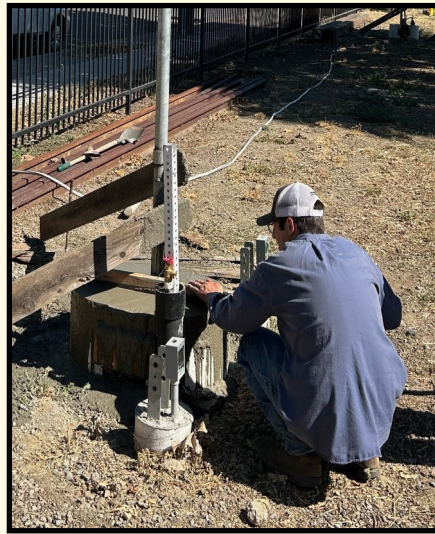
Picnic area light post foundations installed
